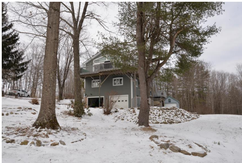
Figure 2 – Photograph showing the exterior of the home at the garage.
